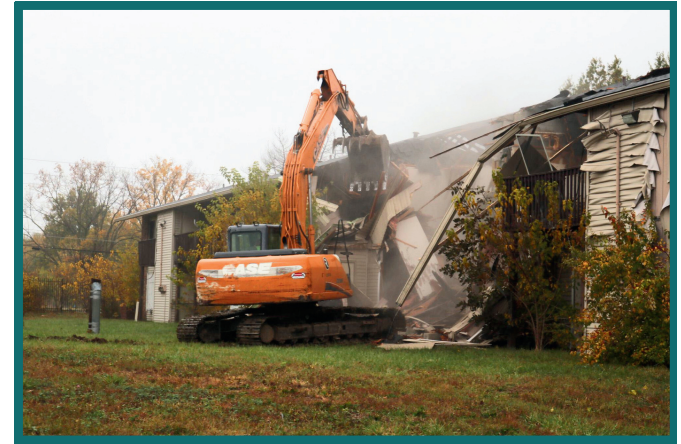
Image: Oaktree Apartments demolition
